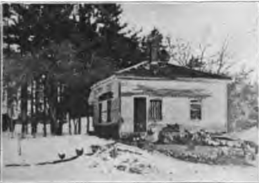
THE OLD NORTH PRIMARY SCHOOL-HOUSE.
